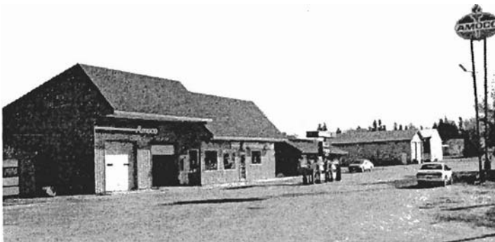
Jeff's Super Service and Y Drive In 1990. (photo courtesy of Eversons)
