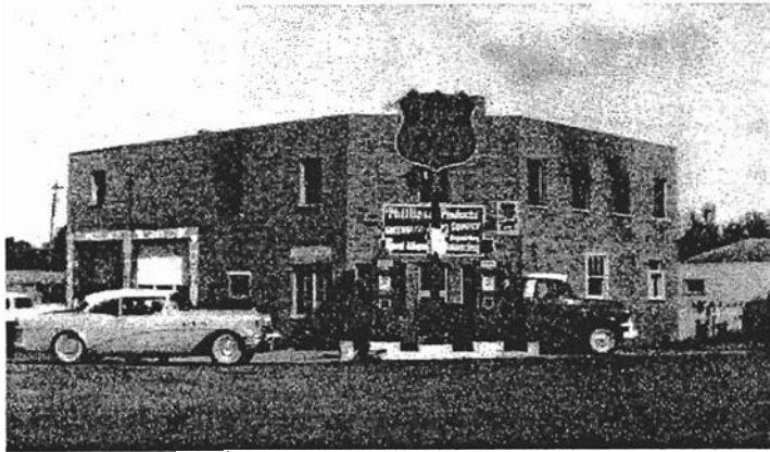
D&F Station exterior after fire June 28, 1958. (Eul/ice)
