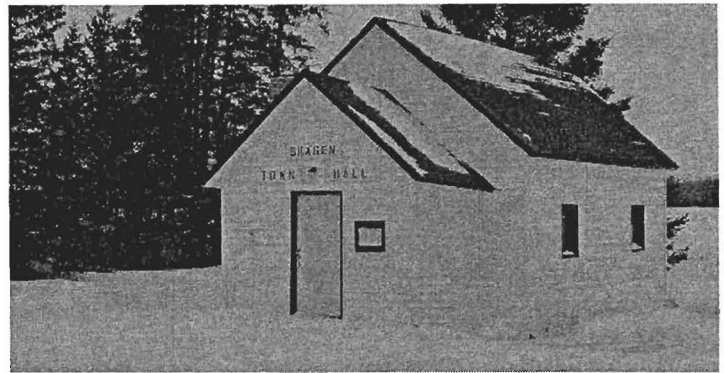
Skagen Town Hall located on County Road 2. (photo courtesy of Karen Janousek)
