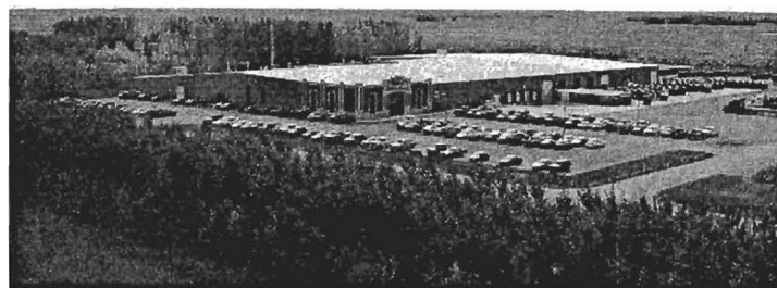
Central Broiler (photo by Central Broiler)
