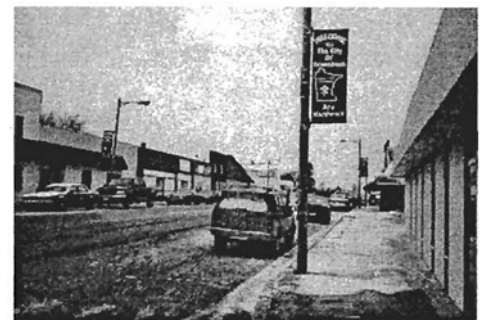
Main Street - Bank to Remedies.
